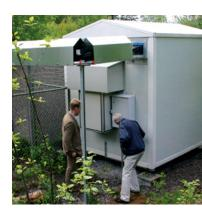
thermal insulation. The cabinets are light, strong and weatherproof, but indoor mounting offers the best protection against weather and vandalism. The units use through-wall air intake and can be wall, floor or roof-top mounted.
